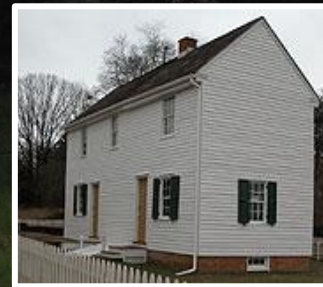
Peter Mott House Underground RR Museum
