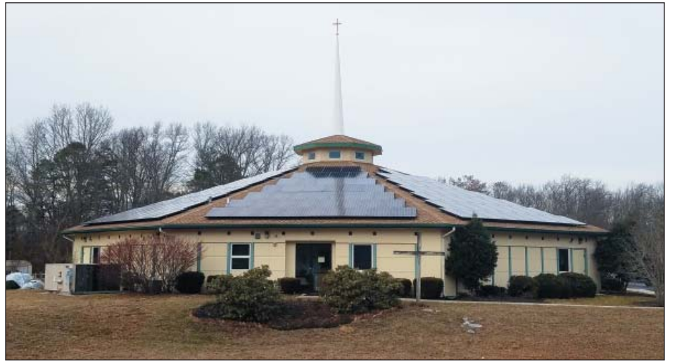
Jackson UMC in Jackson Township has officially gone solar. Photo provided
